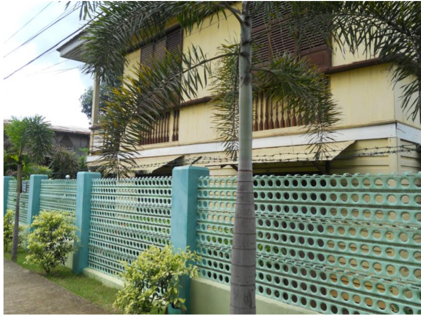
Figure 10. Photo: Donna Amis Davis (used with permission). A residential home in Puerto Princesa, Palawan in the Philippines, rescued and reused mats after the long US military presence in that country (1898-1941, 1944-1991). On Palawan, a local museum also showcases Marston Mats, using them as perimeter walls and as shelving for military artefacts, such as military helmets. Elsewhere, Marston Mats also make up significant sections of the US-Mexico border wall, effectively a military installation, and they have appeared reused in housing after being rescued as “fossil capitalism” from the former Italian Agip (Azienda Generale Italiana Petroli) oil fields on Rig Mountain in Iran (Khosravi 2019). Having underpinned the Normandy Landings, the Berlin airlift and military colonialism in Southeast Asia, Marston Maps now serve a wide variety of other uses, upcycled for good and bad.
